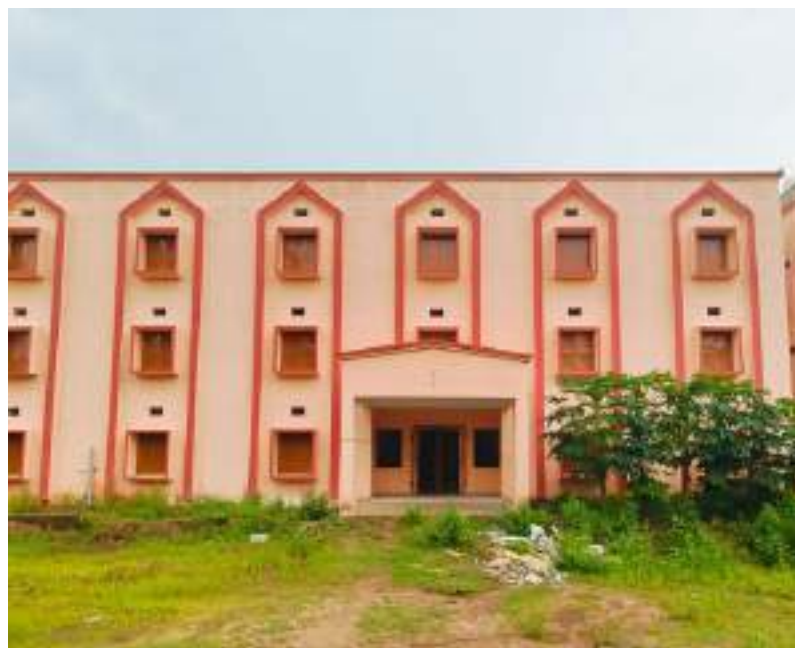
Newly Built 100 Seated ST Girls' Hostel, Bhatangpadar
