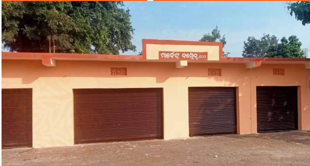
Newly built Market Complex (3) in Sagada | Ready for Inauguration
